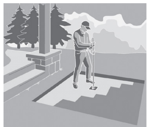
STEP 2: LEVELING AND COMPACTING THE BASE
