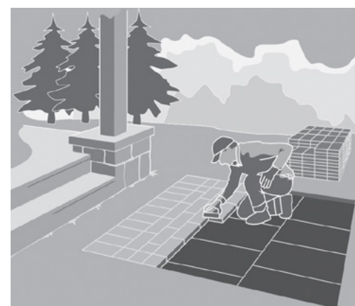
STEP 6: INSTALLING PAVERS
