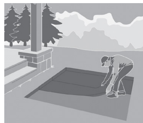
STEP 3: LAYING GEOTEXTILE
