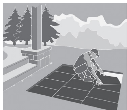
STEP 5: INSTALLING EZ BASE PANELS
